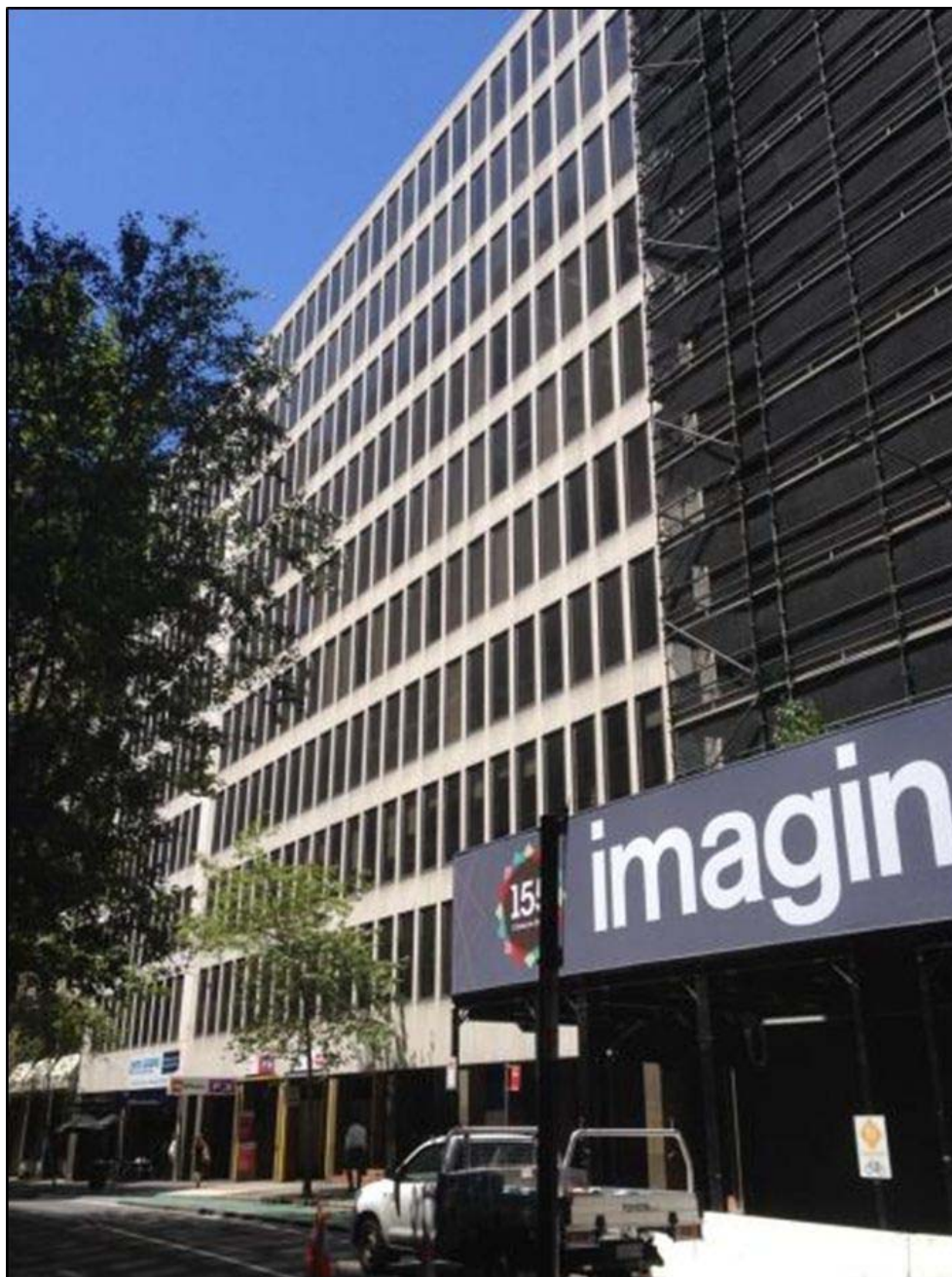
Figure 3: View of the existing building on the site from Kent Street
